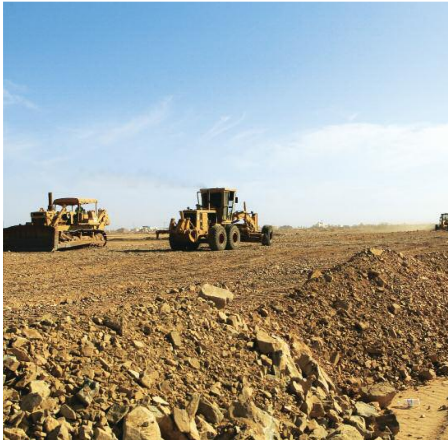
Contractors have been mobilized on site and work is progressing according to the set project program
