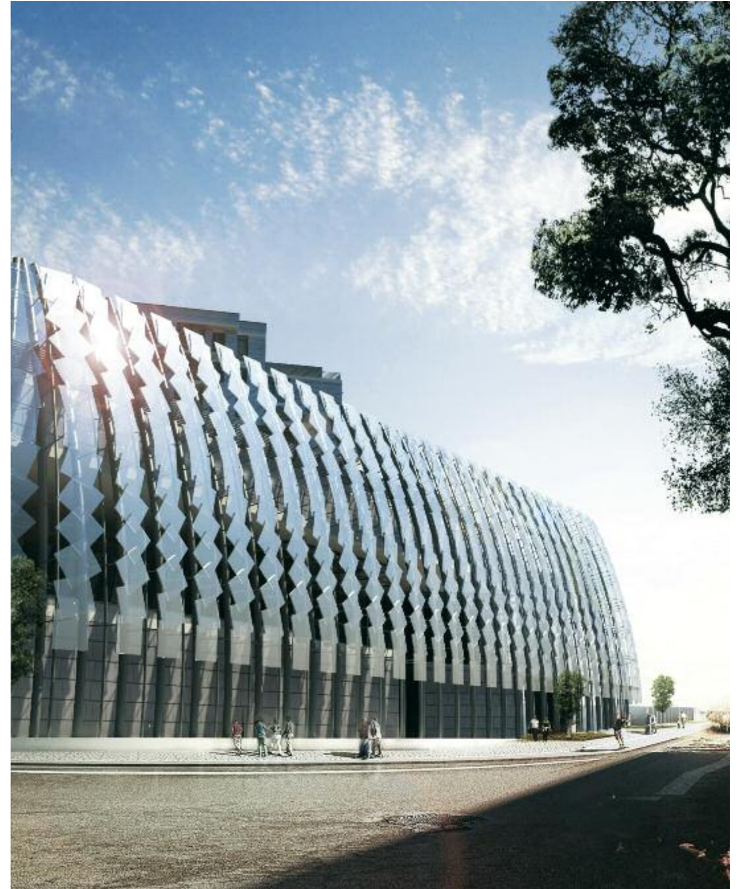
CLUBHOUSE Annexed to the renovated heritage structure that accommodates the clubhouse is a modern structure hosting a number of sports facilities
