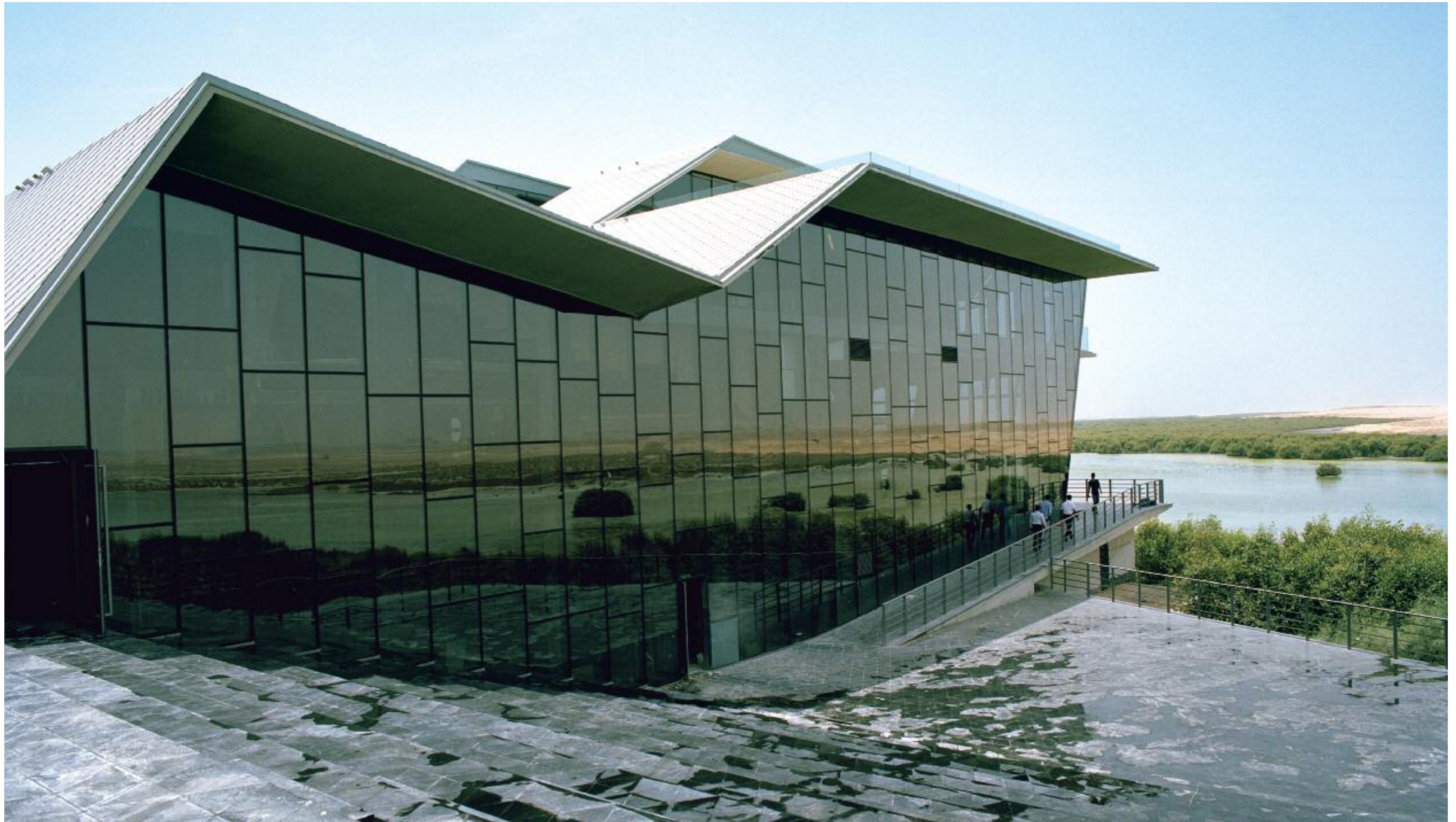
THE PAVILION The Pavilion's folded canopy-like roof is reminiscent of the surrounding topographical strata that drift down to the water
