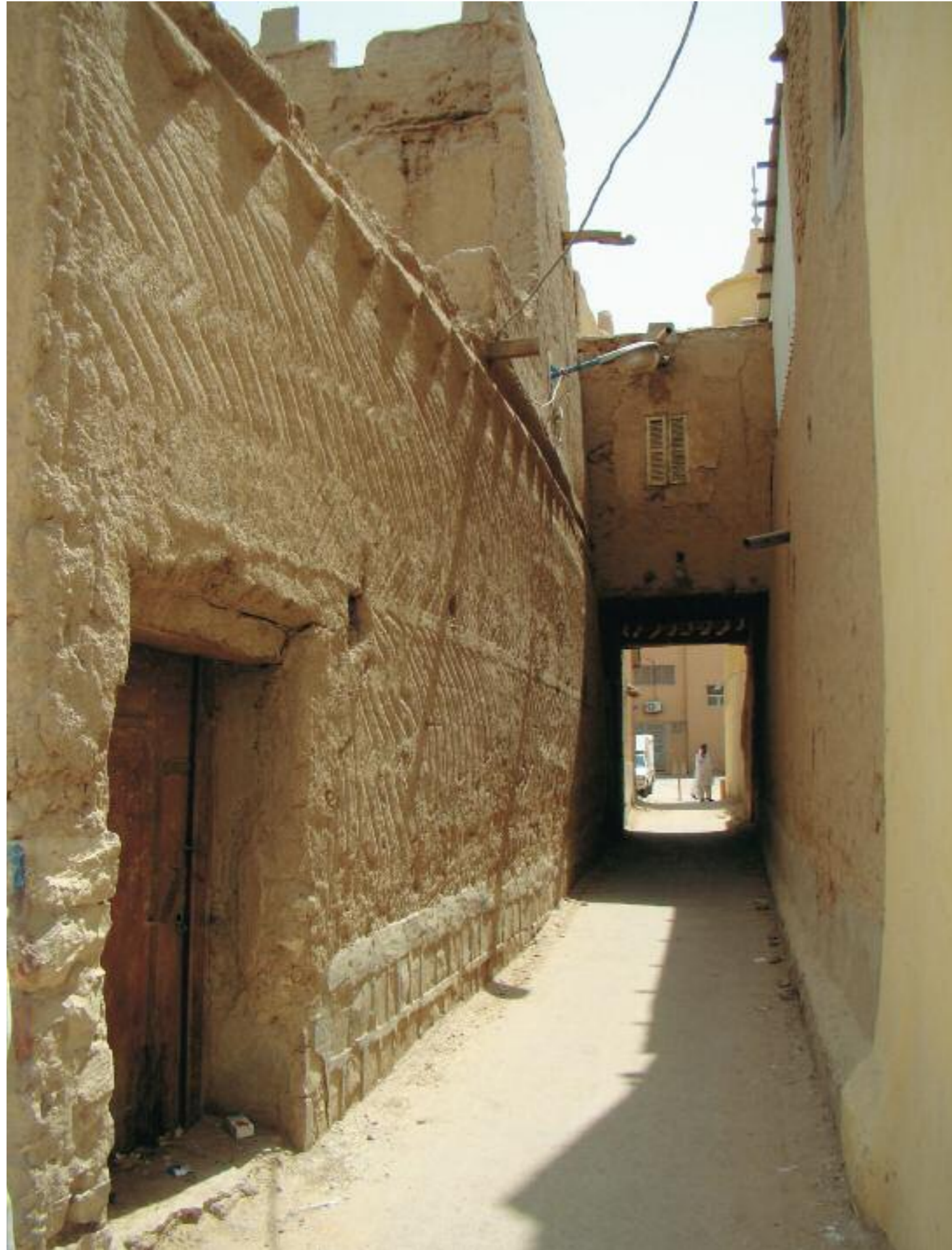
Semi-demolished mud-brick houses within clusters of quiet neighborhoods will be completed with modern infills
