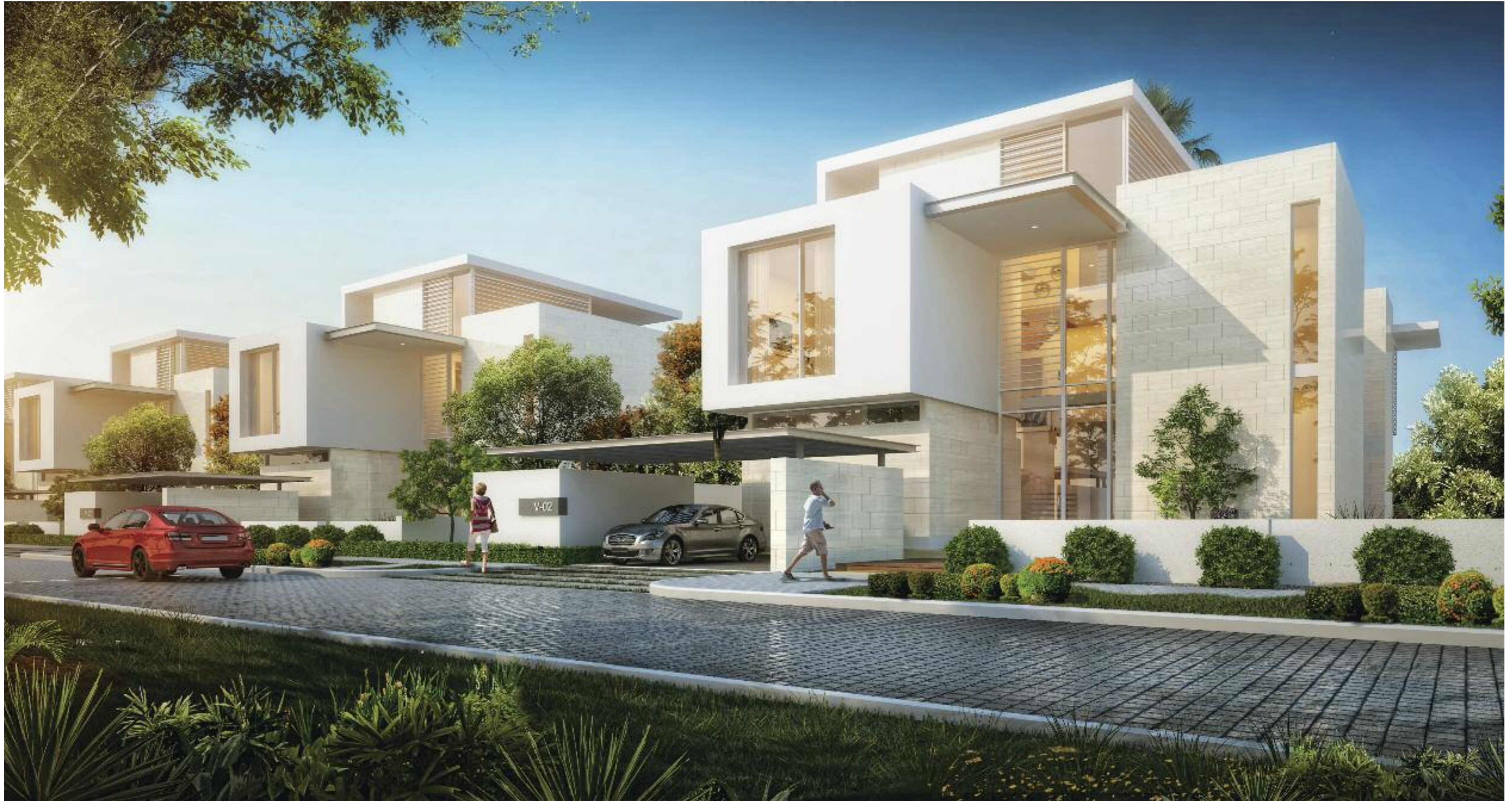
AL ZORAH GOLF VILLAS The two-level villas provide a sense of dynamism and space, with high ceilings in the entrance and lounge areas
